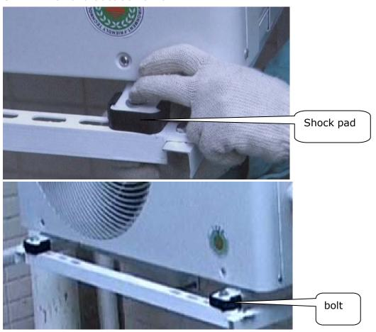
Note: The outdoor unit base must be fixed with the bolts to reduce vibration and noise, if necessary the shock pad can be used.
