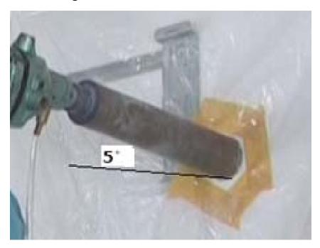
**Note:** The tool need to raise 5 degrees when drilling, so that the hole of the indoor side will be higher than the outdoor side, the water can drain smoothly.
