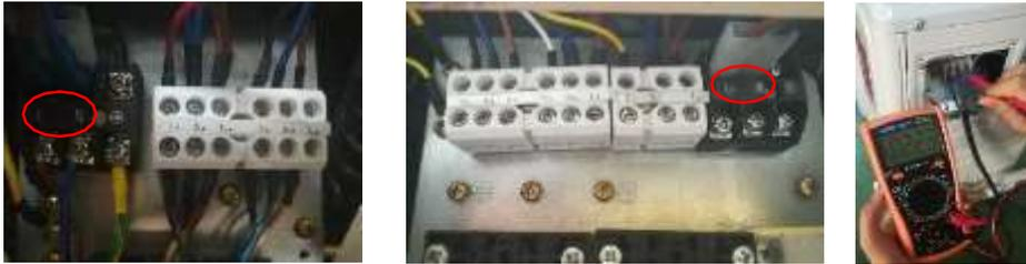
2) If the 1 & N which connect to indoor unit voltage is normal, measure the voltage between the outdoor terminal 1A, 1B, 1C, 1D and N. If the voltage change occurs between 0~24V (change pulse voltage), please replace indoor main PCB.
